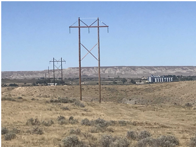
New transmission line for the Iron Creek Substation.
