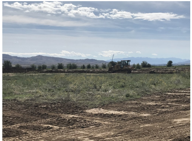
Bulldozing work for the start of Iron Creek Substation.
