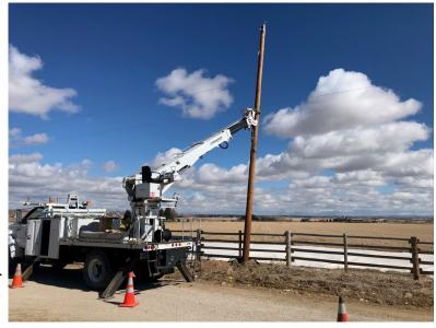
setting the pole. Once the pole is set, depending on what all is on the pole, one to two guys will go up and do the overhead work on the new pole while the others keep an eye on them for safety reasons. At least one guy on the ground is required to keep an eye on the guys in the air.
